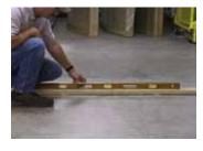
Install frame into opening. Shim frame so that it is plumb, level and square. Attach frame to opening using provided installation screws, No. 10 x 2-1/2" Phillips flat head. Place screws in each of the six (6) pre-punched installation holes. Screws are required to have an embedment of 1-1/2" in wood or 1-1/4" in a masonry structural member. Shims should be placed at all anchorage locations of the jamb to prevent bowing of the frame.
