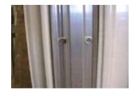
Install door roller track. Before placing roller track in the sill, pre-drill six holes with a 1/8" drill bit—two
