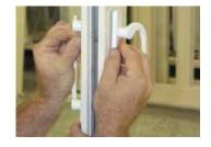
Install the keeper on the astragal of the secondary panel using four (4) - #8 x 1-3/4" pan head truss screws. The top and bottom screws should be installed first, located at the dimple areas. Adjust as needed for the lock to work properly and then install the remaining two screws.
