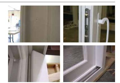
Install pre-cut 4 1/2" bumper stops in interior track of head and sill. Caulk where the panel stop meets the side jamb at the sill.
