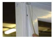
After the fixed panels are in place, drill 1/8" pilot holes into the weather-strip track starting 6" from each end, with a maximum 12" spacing between the remaining screws. The drill bit needs to be a minimum of 4" in length to prevent damage to the frame. Install #8 x 7/8" self-drilling screws with a #6 flat head into each pilot hole.
