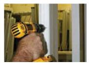
Install the multi-point mortise latch into the cutout located in the edge of the primary operating panel (without the astragal), using two (2) - #8 x 3/4" flat head screws. Make sure the holes in the face of the panel line up with the receivers for the handle set before fastening the mortise latch to the panel.
